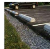
Figure VFS-2 Vegetated filter strip between parking lot and street. San Antonio River Authority. Photo source: Telsa Tech, Inc. Rendering components: San Antonio River Authority. University Department of Biological and Agricultural Engineering. Source: Telsa Tech.
