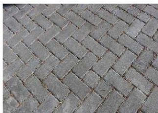
Figures PP-1 and PP-2 Permeable parking installations at the San Antonio River Authority Guarneri Offices (bottom) and at Confluence Park.
