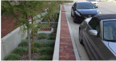
Figure HFM-2 High-flow Media BMP including surface vegetation adjacent to street in San Antonio. Source: HART Associates, Inc.
