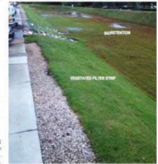
Figure TTVFSBR-1 Vegetated filter strip surrounding a bioretention area in a parking lot, Raleigh, North Carolina. Source: TerraTech, Inc.
