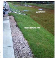
Figure TTVFSBR-4 Vegetated filter strip surrounding a bioretention area in a parking lot, Raleigh, North Carolina. Source: TerraTech, Inc.
