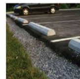
Figure VFS-2 Vegetated filter strip between parking lot and stream. San Antonio River Authority. Photo source: Telsa Tech, Inc. Rendering components: San Antonio River Authority. University Department of Biological and Agricultural Engineering. Source: Telsa Tech.
